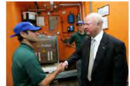
Energy Secretary Bodman views the hydrogen energy storage system
